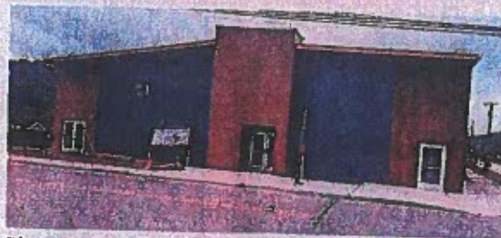
The exterior of the new Black Diamond Brewery and Distillery, in partnership with Hocking College, will soon have a Black Diamond sign once construction is complete.
